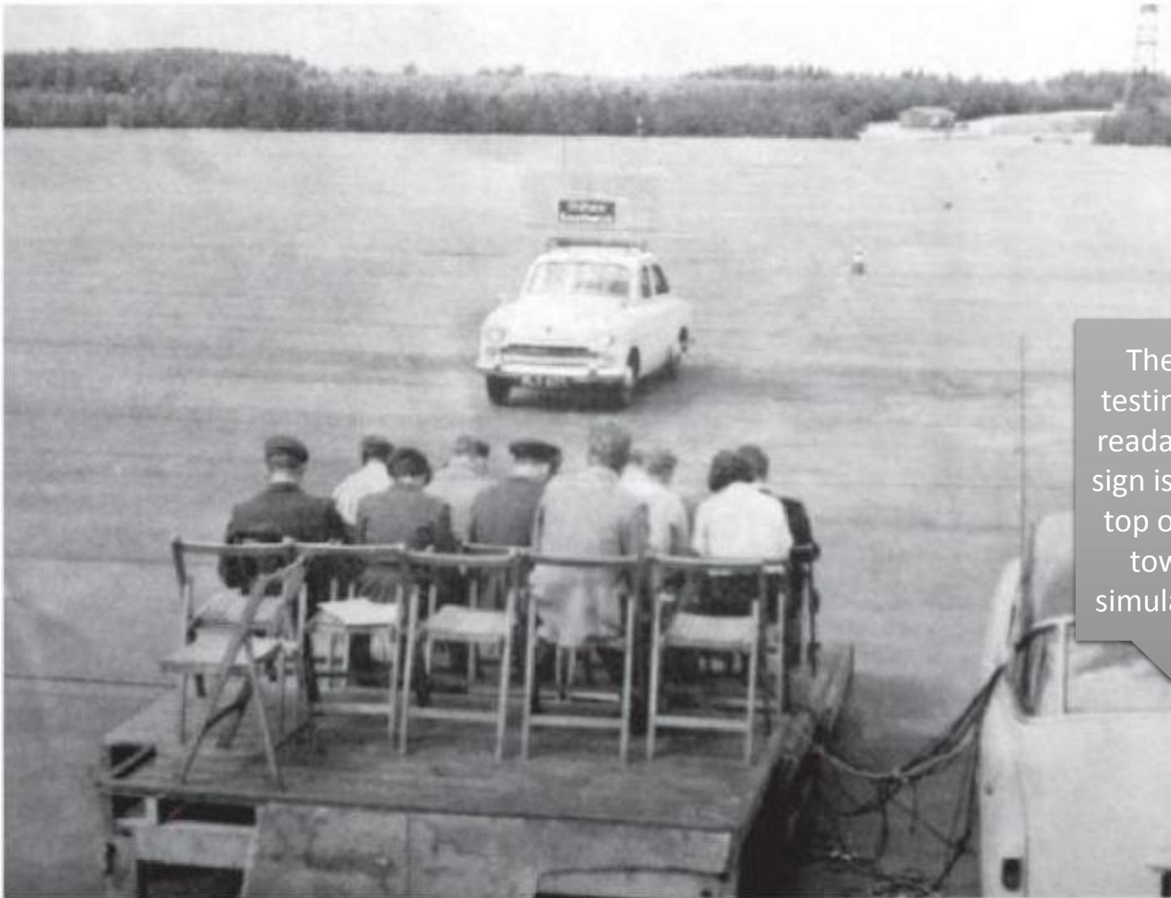
These people are testing road signs for readability – the road sign is being driven on top of a car at speed towards them to simulate roadway use
