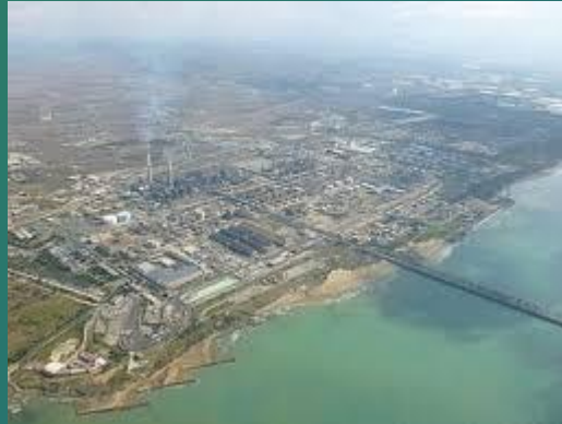
Petrochemical plant – Gela, Italy
